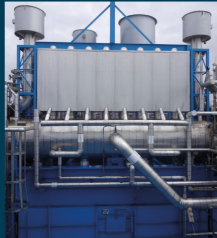
Secondary steam separation in bottles outside drum
